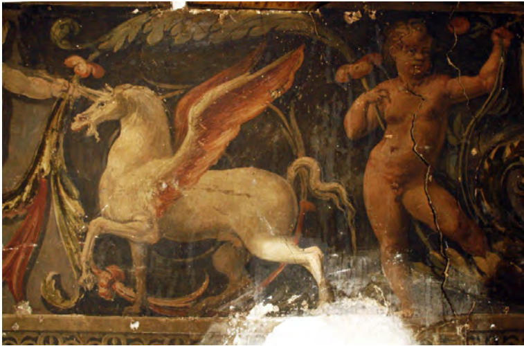
Figure 15. Details of the ancient restoration below the left beam.
