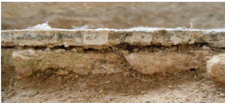
Figure 4. In situ detachment of the tessellatum and its bedding layer from the nucleus.
