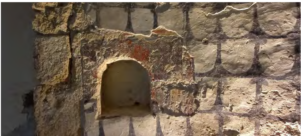
Figure 3. Concattedrale of Santa Maria Assunta in Venafrò (IS) displaying a palimpsest of fresco paintings from the 5 th , 13 th , and 15 th centuries. The noticeable lack of adhesion between the renderings has resulted in significant loss and lacunae.
