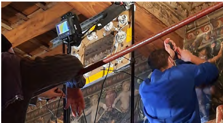
Figure 21. Thermography set during the consolidation (it is visible the thermocamera and the frame with halogen light).
