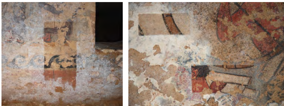
Figure 23. Cleaning tests with the removal of calcite depositions. (Left) north-west wall and (right) south-east wall of the tomb.
