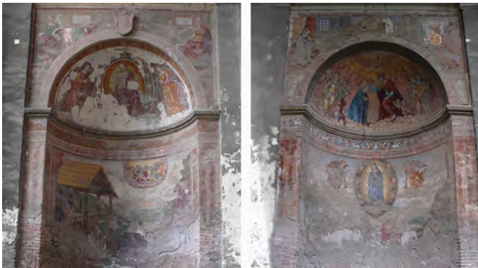
Figure 7. South chapel (on the left) and west chapel (on the right) of the church S. Maria delle Fortezze. Viterbo.
