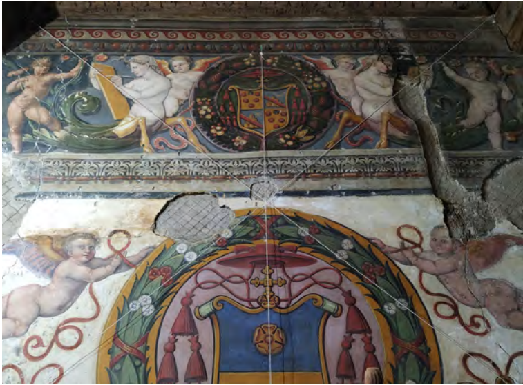
Figure 11. Strings stretched from the fireplace's frame to the beams. One can observe the construction lines of the painting. Just below Ridolfi's emblem, the points marked in correspondence of the string.
