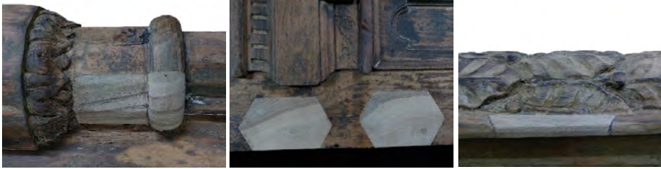
Figure 13. Partial repair with new wood (Photo. I. Özsaıt-Kocabaş)
