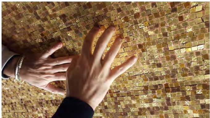
Figure 7. Auscultation by tapping with the fingertips.
