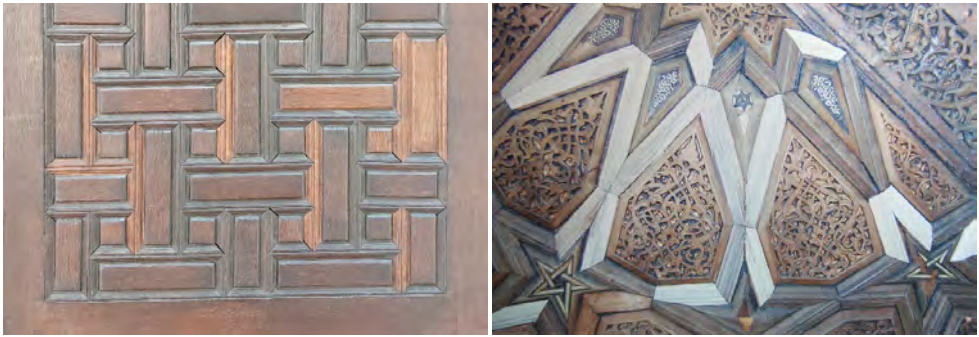
Figure 14. Partial repair on doors with rectangle and star kunderkari composition (Photo. C. Beşiktaş)
