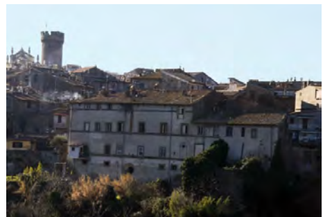
Figure 2. The facade of the palace on the valley.
