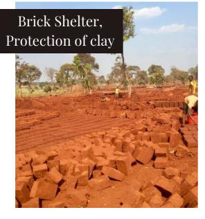
Bricks are often sun-dried, such as in Tanzania, where lime has been added to the clay bricks as a stabiliser to steadily harden the bricks over time.
